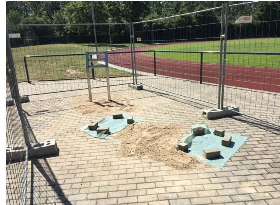
Preparations for the smartbench installation in our school yard.
